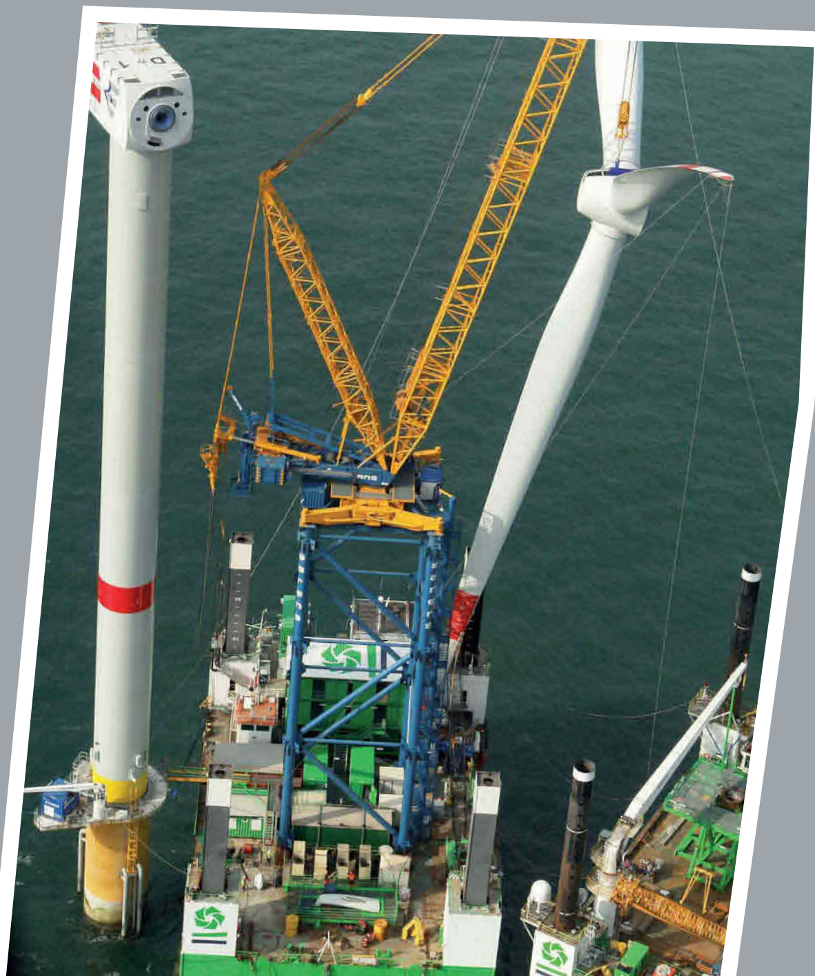
Offshore installation of a wind turbine, Belgium
