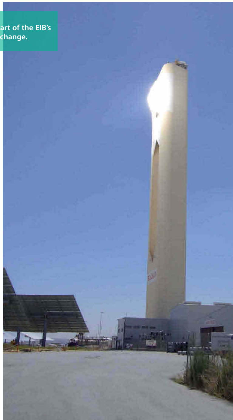
Power tower plant – Solucar, Spain
