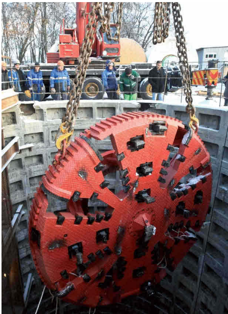
Building of the main collector, St Petersburg, Russia
