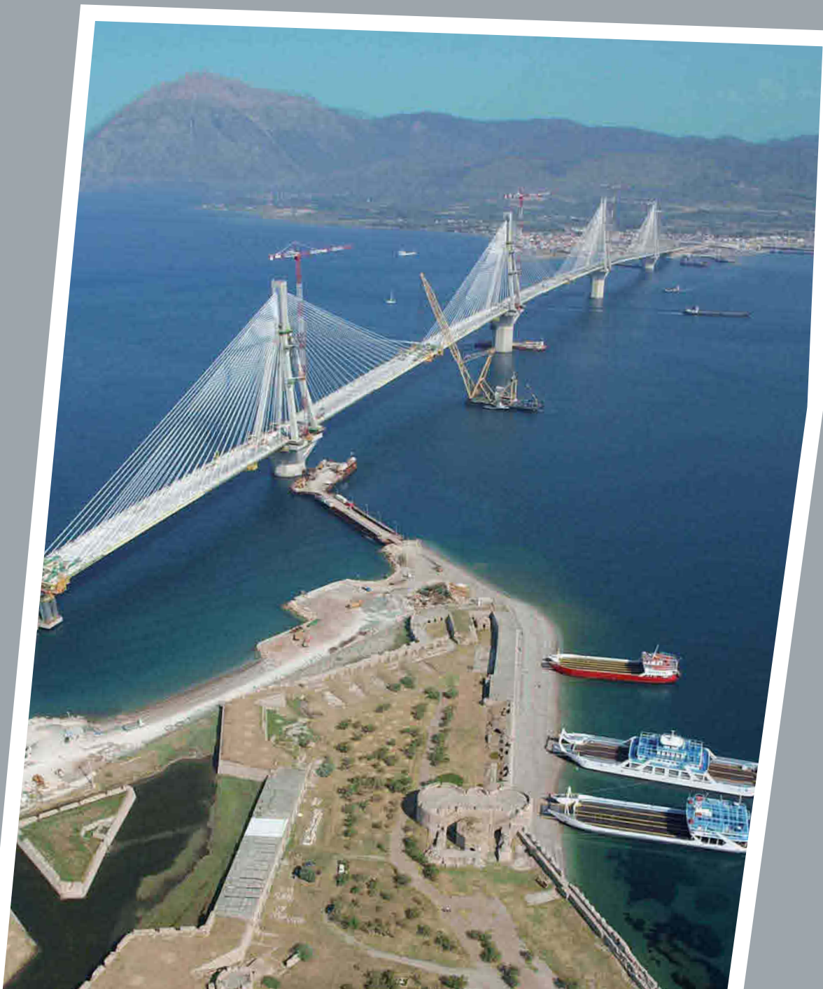
Rion-Antirion bridge across the Gulf of Corinth, Greece
