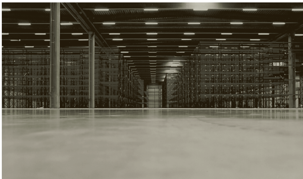
Construction of logistics facilities, Romania
