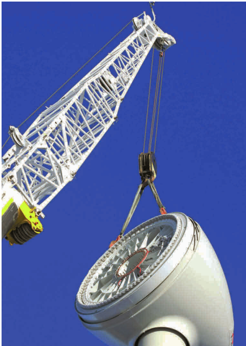
Construction of wind farm
