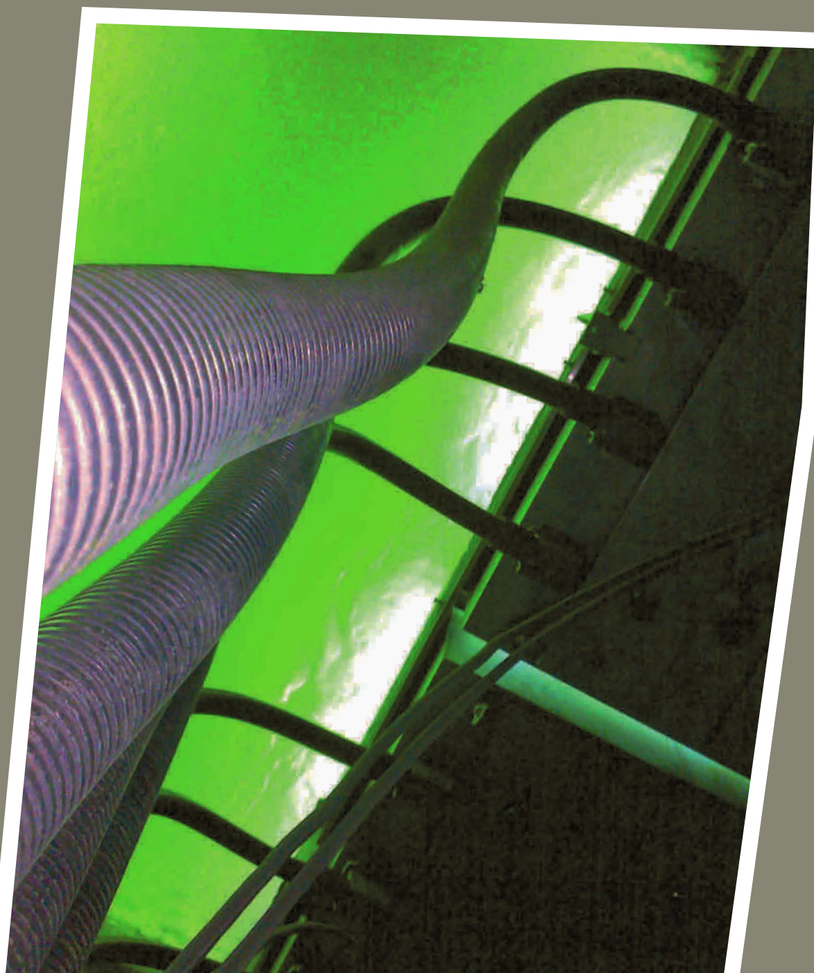
UV disinfection channel, south-west wastewater treatment plant, Saint Petersburg, Russia
