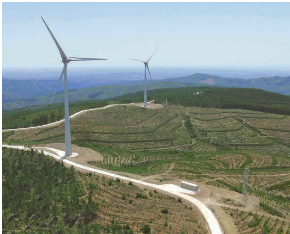
Mougueiras wind farm, Portugal
